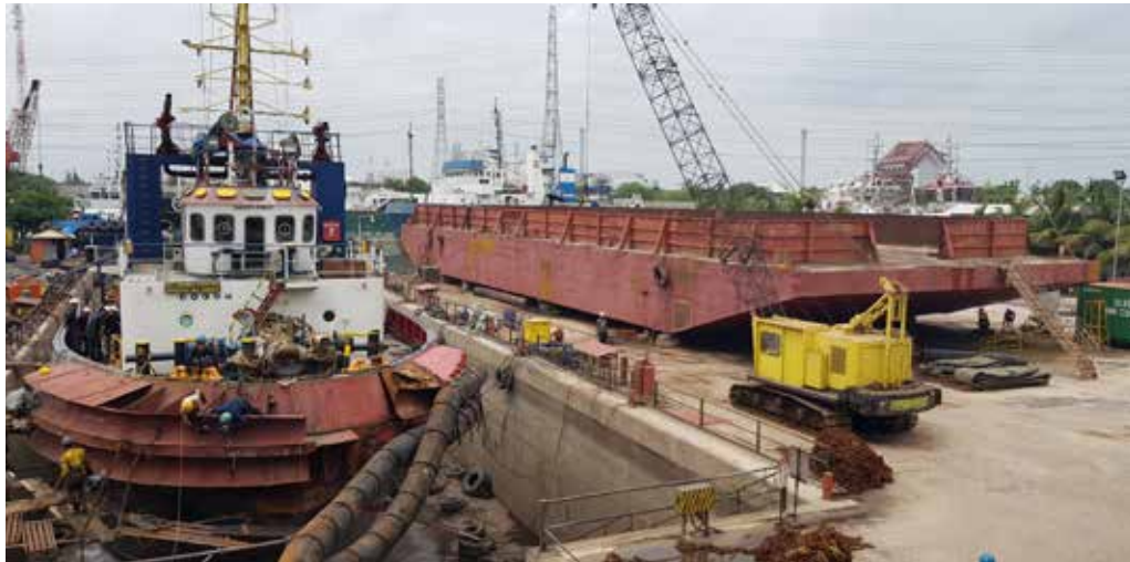
GRAVING DOCK I
