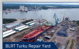
BLRT Turku Repair Yard
