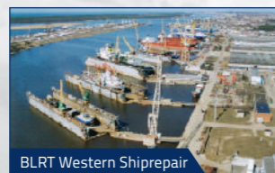
BLRT Western Shiprepair
