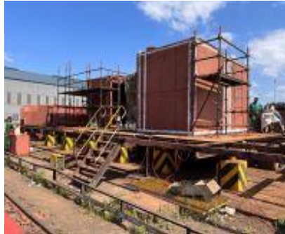
2 x BWTS Deck under construction
